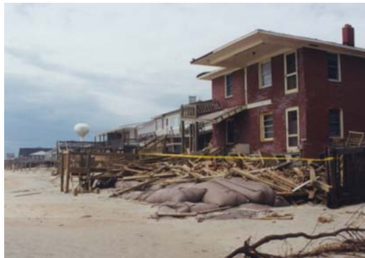
Sandbags protecting a home near 4 th Street, Emerald Isle days after hurricane Floyd in 1999.
