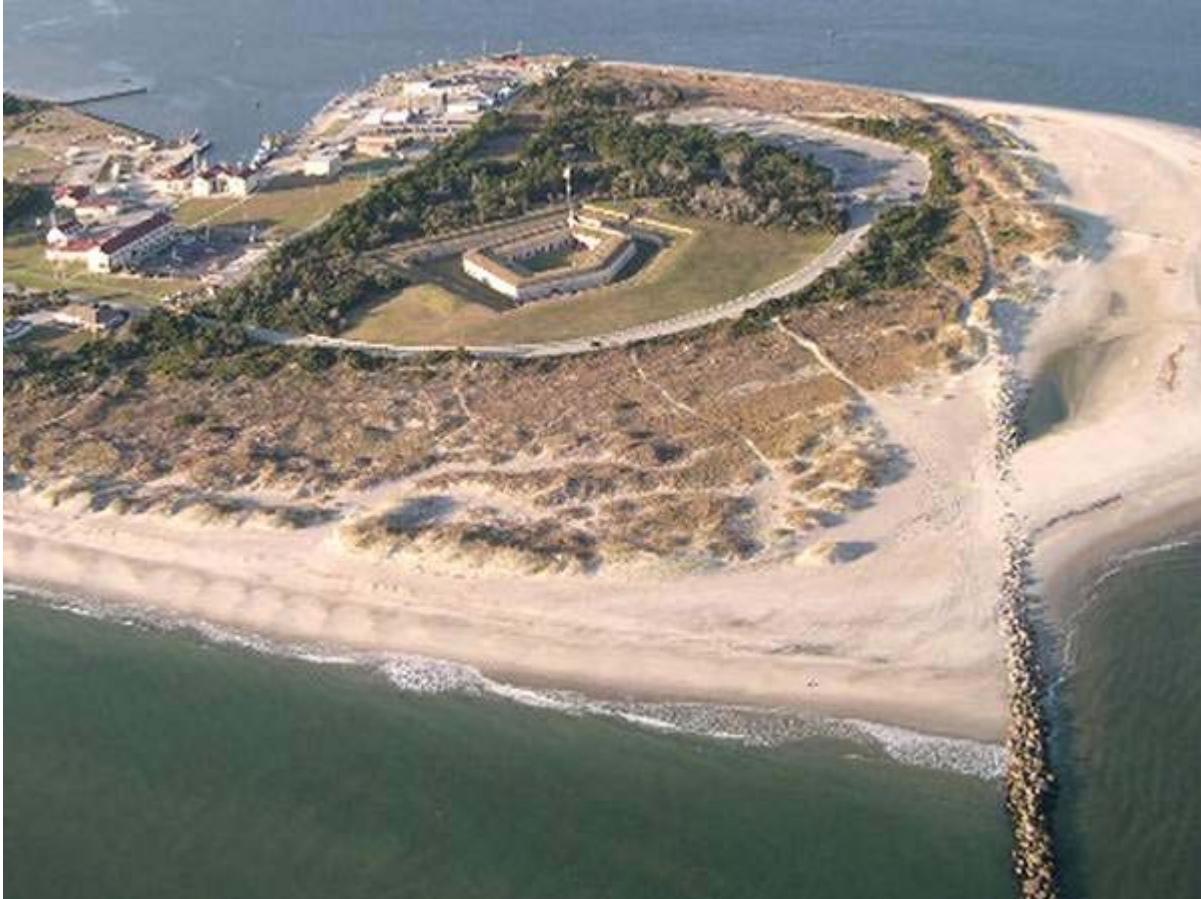
The structure at the east end of Ft. Macon State Park on Bogue Banks is considered as one of two "terminal groins" in the State. The other is situated along the north end of Pea Island on the Outer Banks, and helps protect the Bonner Bridge over Oregon Inlet.
