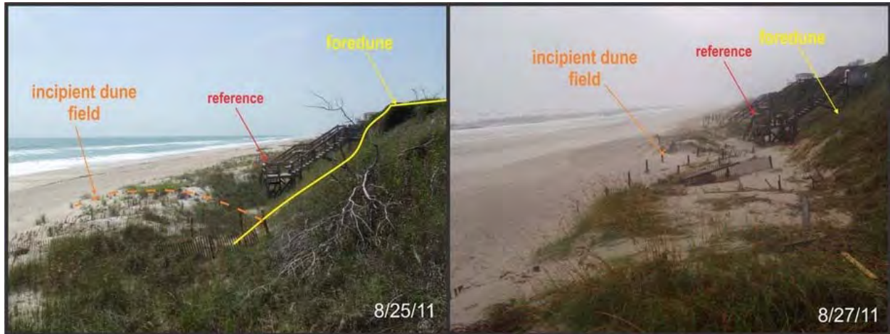
Fig. 2 – “Before” (left panel) and “after” (right panel) from Memorial Park, Pine Knoll Shores. Notice the remaining sand fence posts and absence of sand and fencing slats between the posts on 8/27/11.
