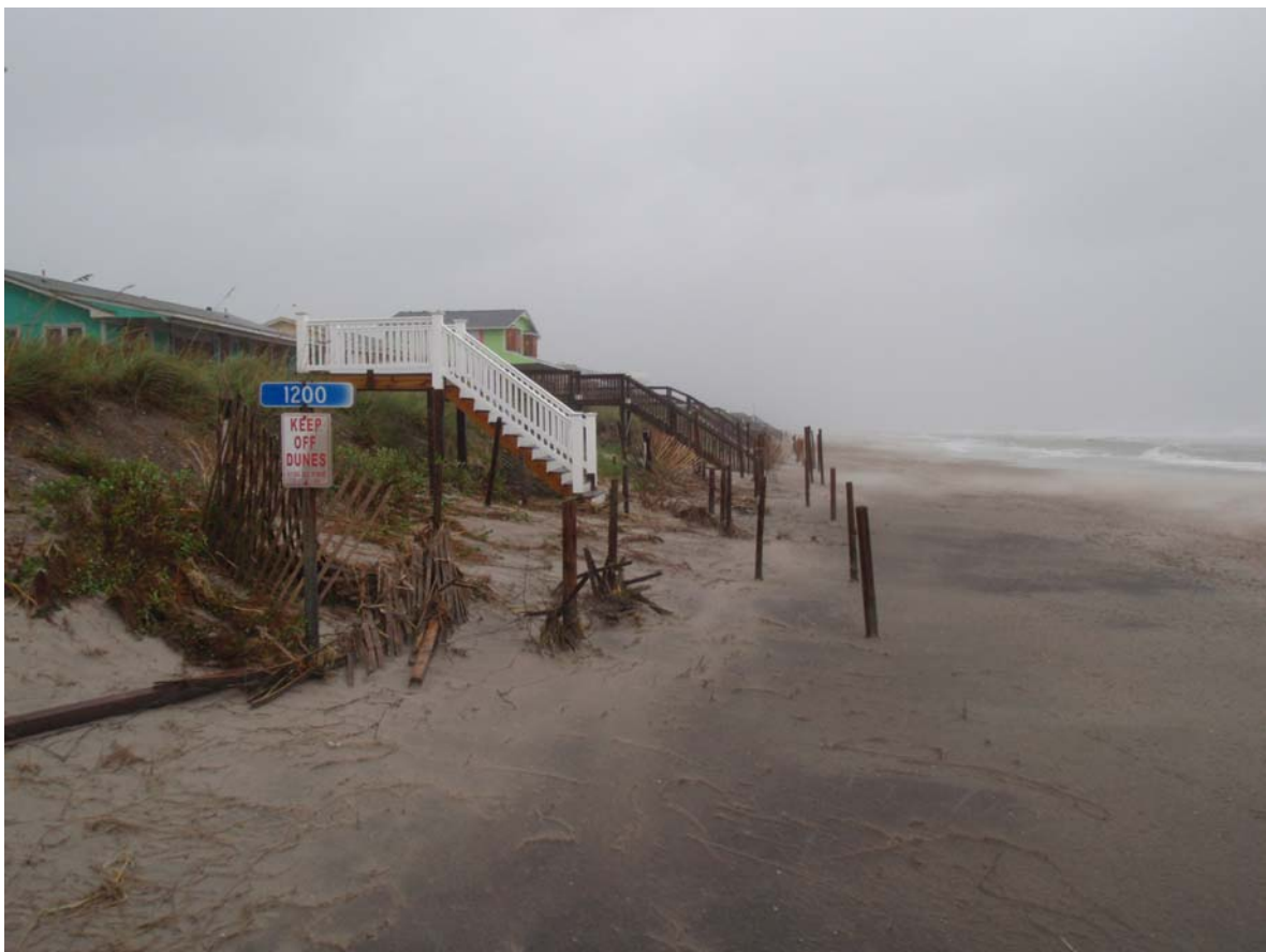
Fig. 3 – 12 th Street, Emerald Isle looking east – “worse” incipient dune erosion.
